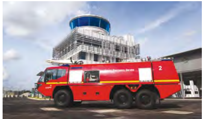
AES shifted into a brand new fire station at Seletar Airport in January 2012.
