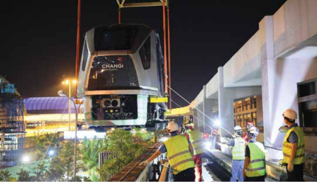
Left: Workers concentrate on aligning the new train car to the tracks, to ensure successful delivery of the new batch of Skytrains.
