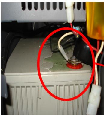
Leakage of Electrolyte from another UPS within the premises probably due to poor maintenance
