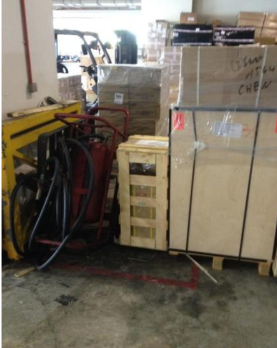
Obstruction to fire extinguisher
