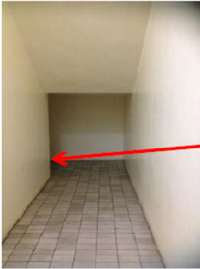
Staircase landing, B16-STR-01
