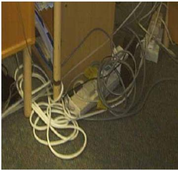
Use extension cords and expansion plugs for temporary wiring only and consider having additional circuits or outlets added by a qualified electrician.
