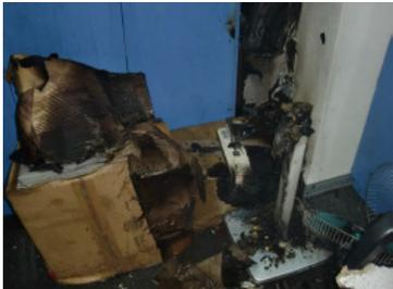
Combustibles such as newspapers and cardboard boxes should not be placed near electrical equipment to reduce fire incidence and spread.
