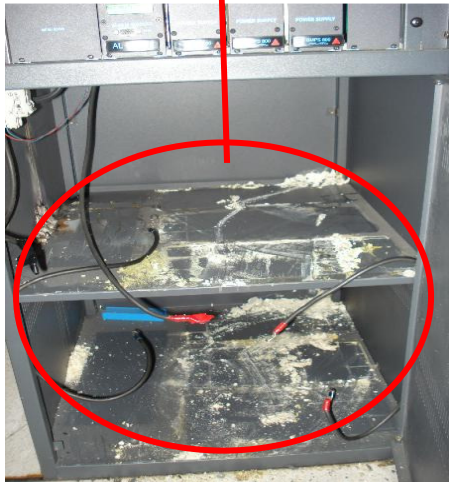
Residues of electrolyte found within the UPS cabinet
