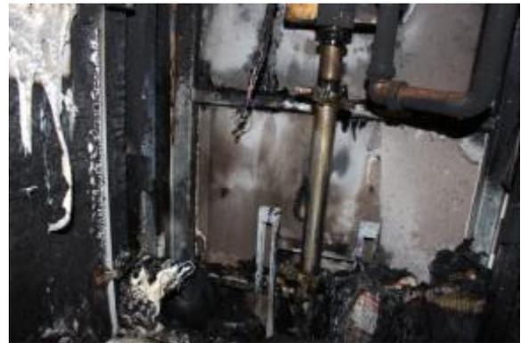
Figure 2 – Burned cabinet within service duct
