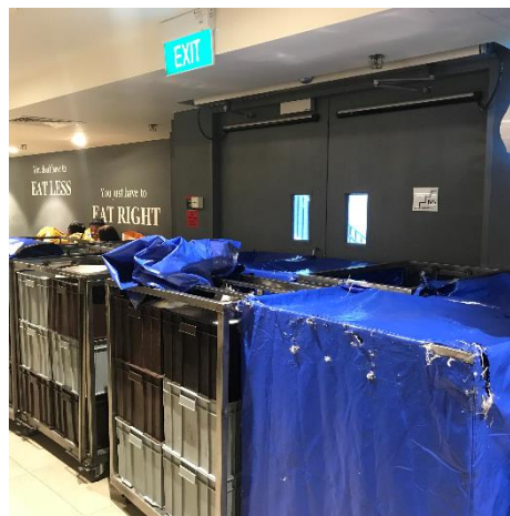
Pic. 2 – Obstructed Evacuation Exit
