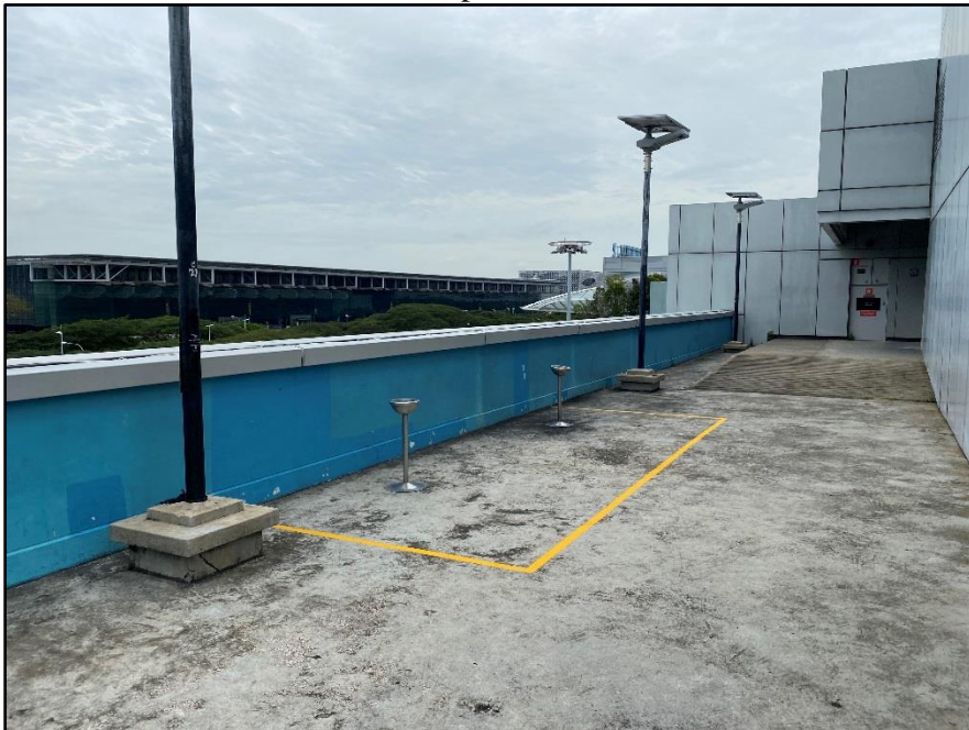
Terminal 2, South, Level 3M, Carpark 2A Roof
