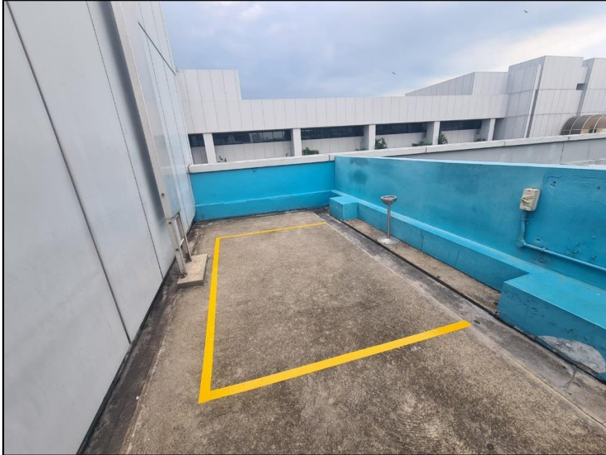
Terminal 2, North, Level 3M, Carpark 2B Roof
