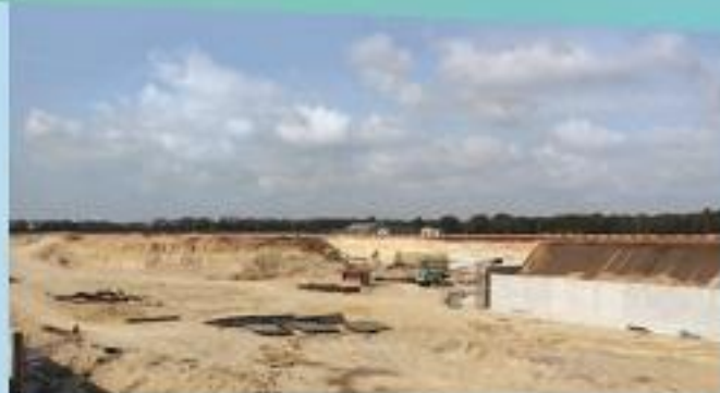
THE NEW RESERVOIR BEING CONSTRUCTED. ITS WATER HOLDING CAPACITY WILL BE THREE TIMES LARGER AND FITTED WITH PUMPS FOR BETTER FLOOD PREVENTION
